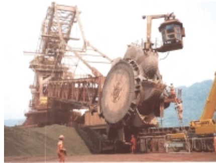
Figure 1: Mounting the replacement gear on the Brazilian bucket-wheel excavator
