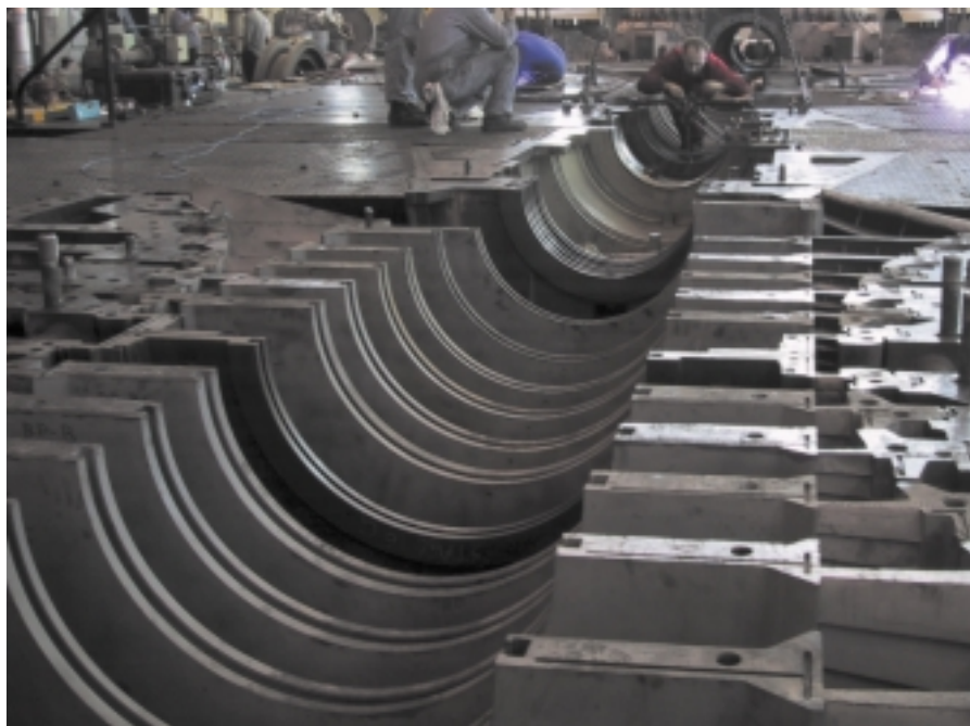
View of open steam turbine (TopsOff)
