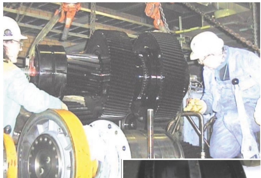
Fig. 3: Dismantling the intermediate shaft
